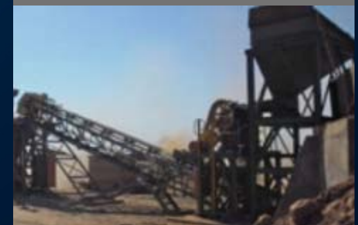
CRUSHING PLANT - DIAMONDS, ZIMBABWE
