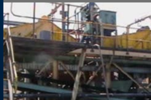
350 000 TPA DMS PLANT - GOLD RSA
