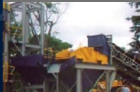
ALLUVIAL GOLD PROCESSING PLANT - WEST AFRICA
