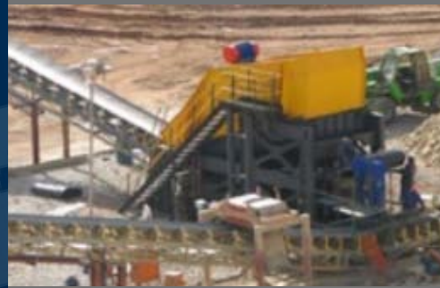
7 000 000 TPA SCREENING PLANT - AFRICA
