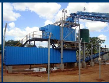
Construction of a 2 300 000 tpa Process Plant 65 tph Dense Medium Separation Plant Screening Plant X-Ray Recovery
